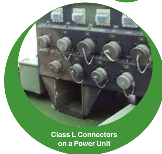
Class L Plug and Receptacle
